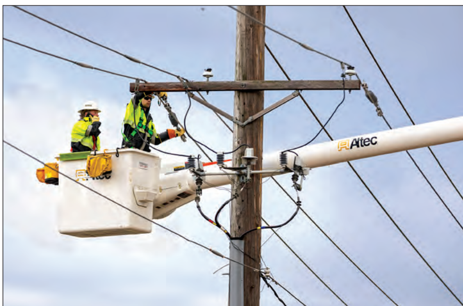
Ayrton Breckenridge/The Daily Iowan MidAmerican lineworkers fix electrical lines alongside Highway 6 after a tornado went through parts of Coralville on Friday. The Coralville fire and police departments worked alongside other agencies to help facilitate cleanup.
