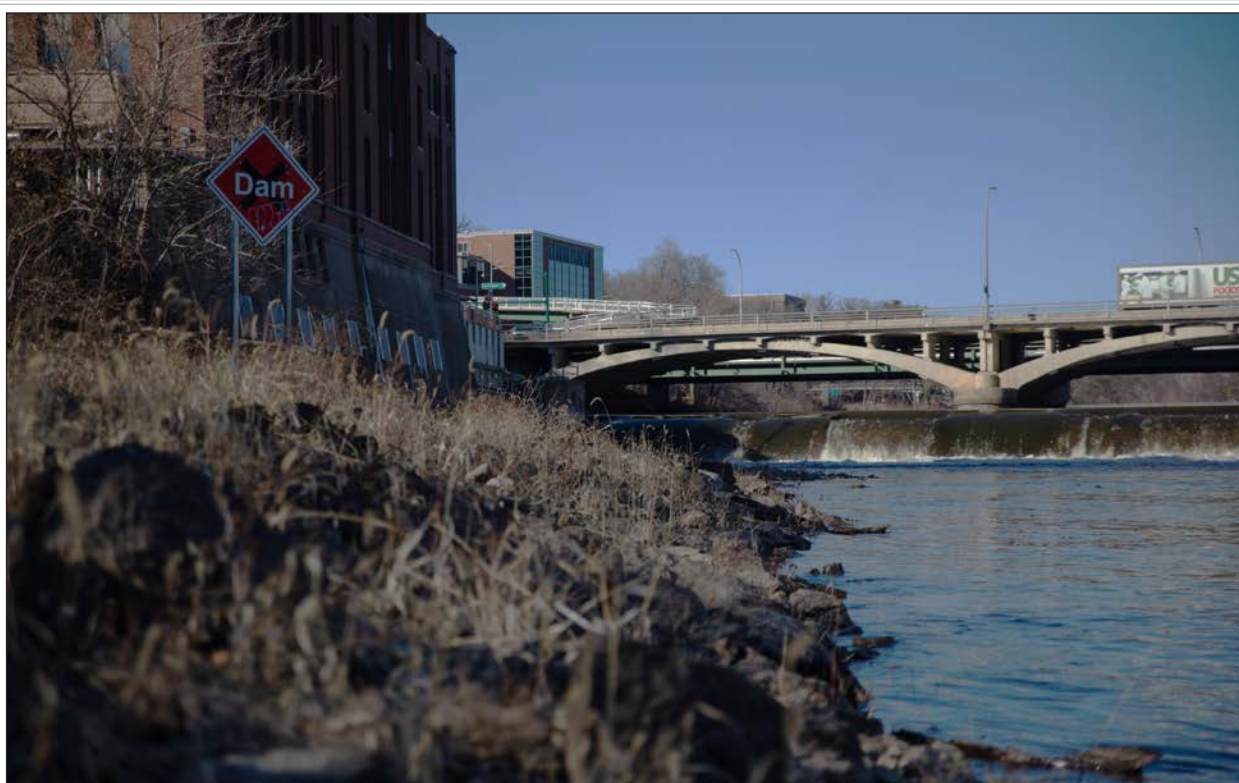
The Burlington Street Dam on the Iowa River is seen on Feb. 13.
