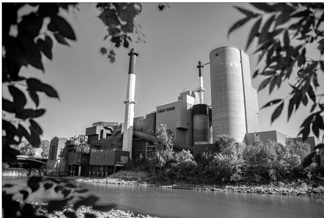
The University of Iowa Power Plant as seen on Oct. 19, 2021.
