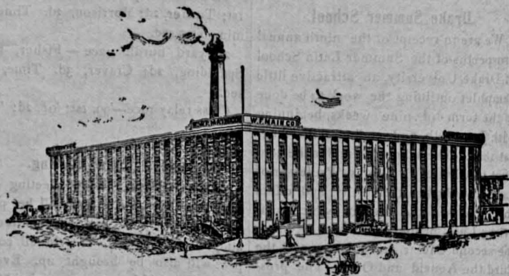
THE W. F. MAIN CO. FACTORY UNDER PROCESS OF COMPLETION AT IOWA CITY, IOWA. When Completed will be the Largest Jewelry Factory in the United States (containing over 35,000 feet of floor space) and the only one Located in the West.
