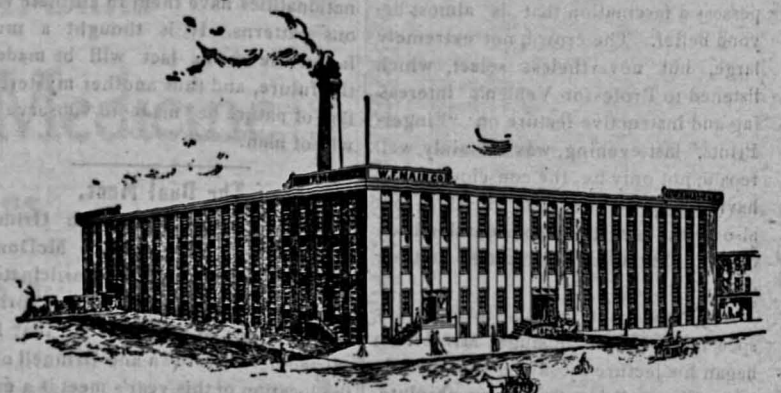
THE W. F. MAIN CO. FACTORY UNDER PROCESS OF COMPLETION AT IOWA CITY, IOWA.
