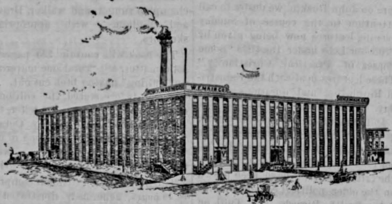
THE W. F. MAIN CO. FACTORY UNDER PROCESS OF COMPLETION AT IOWA CITY, IOWA.
