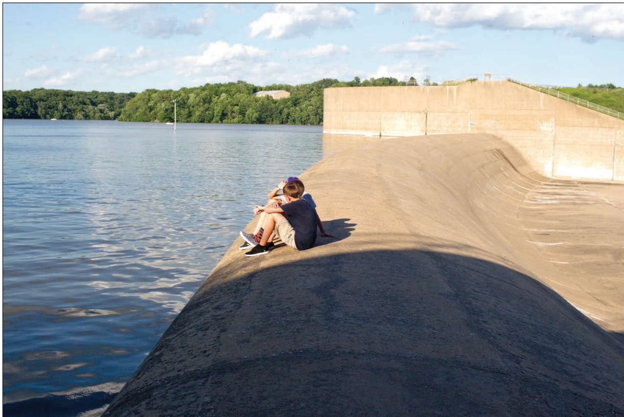
Jonah Wakel and a friend look at the water in the Coralville Reservoir from the dam's emergency spillway. The spillway has not been topped since the 2008 flood. (The Daily Iowan/Sergio Flores)
