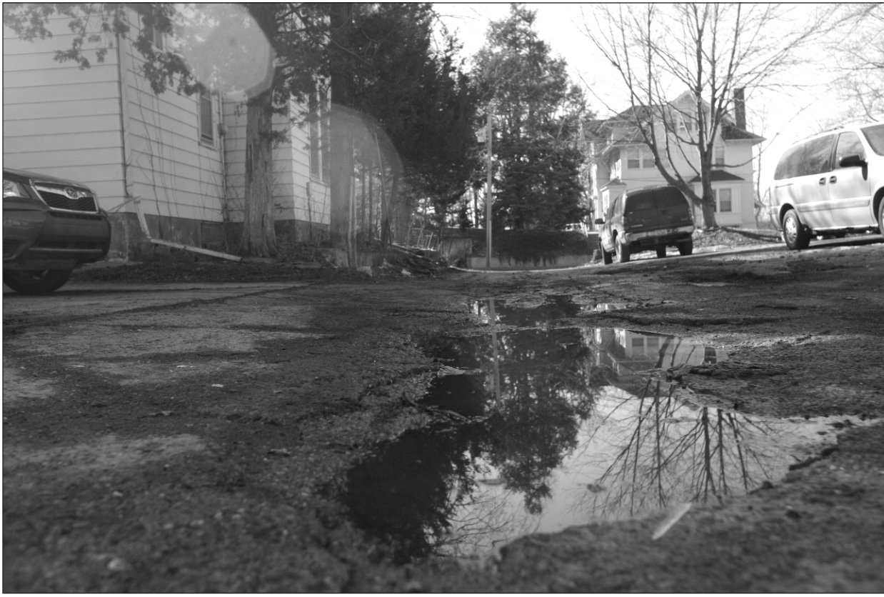
Potholes line an alleyway in between Church Street and Ronald Street in on Thursday. Iowa City is planning on filling 200 to 300 potholes a day. (The Daily Iowan/Margaret Kispert)
