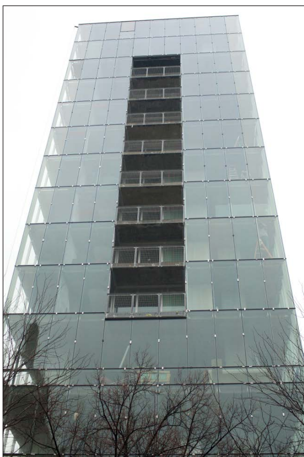
Construction on Park@201 continues on Nov. 20, 2013. The project is reportedly over budget and behind schedule. (The Daily Iowan/Margaret Kispert)
