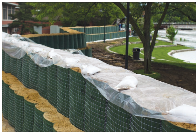
The floodwall behind the IMU is constructed as the river tops its banks on May 31. The floodwaters reached the floodwalls but did not cause major damage. (The Daily Iowan/Joshua Housing)
