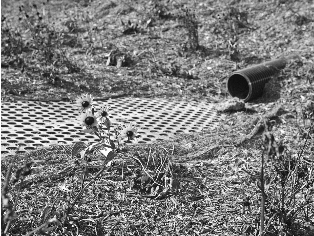
A drain at the bio-retention cell at the Oakdale Campus on Thursday. The rain-garden system is designed to store and filter rainwater before it drains into the Iowa River. (The Daily Iowan/Carrie Guenther)
