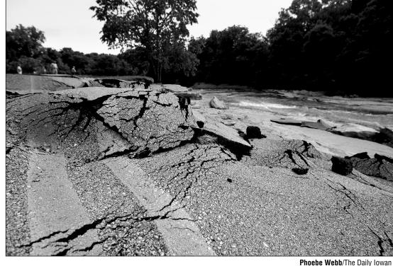
The road at the base of the Coralville Dam spillway is washed out near the Fossil Gorge on Monday. The road buckled under the force of the flood.
