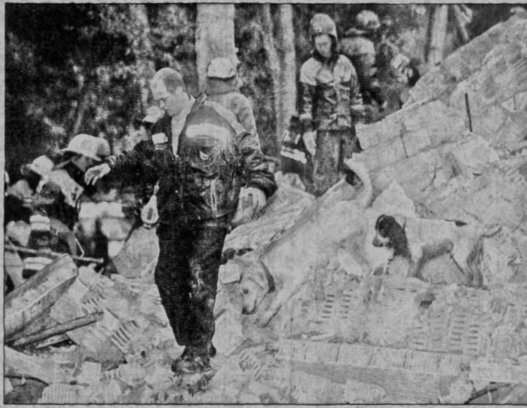
Tatiana Makeyeva/Associated Press A Ministry of Emergency Situations officer with sniffer dogs hunts for survivors at a site of the blast in Moscow Monday. A suspected bomb demolished a large apartment building, leaving 73 people dead and scores of others missing.
