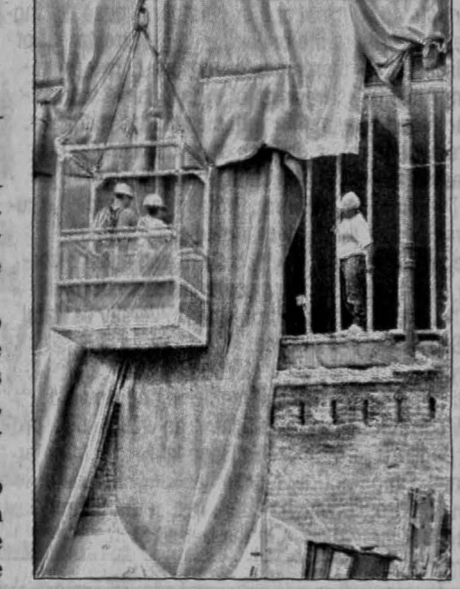
Workers tear down a wall of the Savings and Loan Building.
