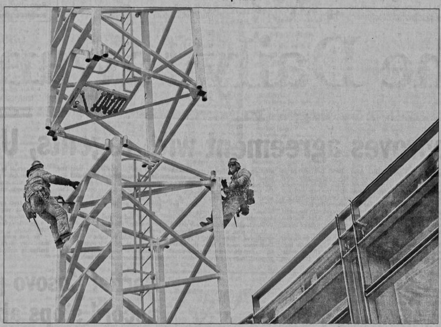
Two workers hold on after disconnecting a 14,000-pound section of a crane at the construction site of the Biology Building. The crane has been up for 13 months; it is being
