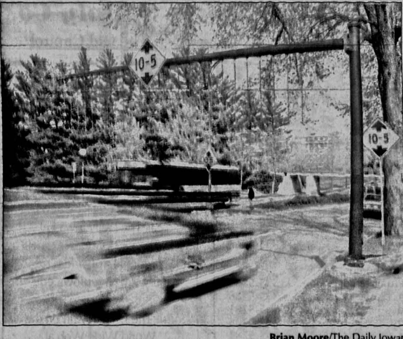
Numerous accidents under the Iowa Avenue bridge have prompted the City to install chains warning drivers of the low bridge clearance.
