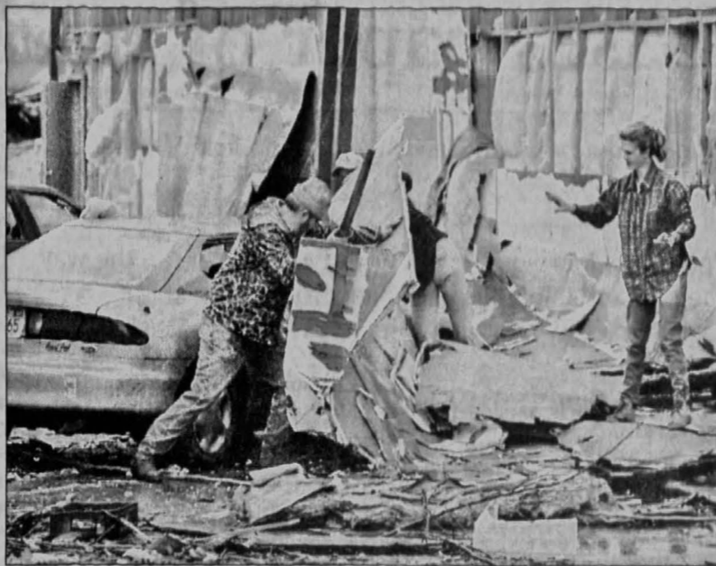
Ken Lancaster (left) and Brian Brown remove wreckage from Robin Fannin's car as she watches (right) Sunday morning. Fannin was at work when a tornado blew apart many of the buildings in downtown Arkadelphia.
