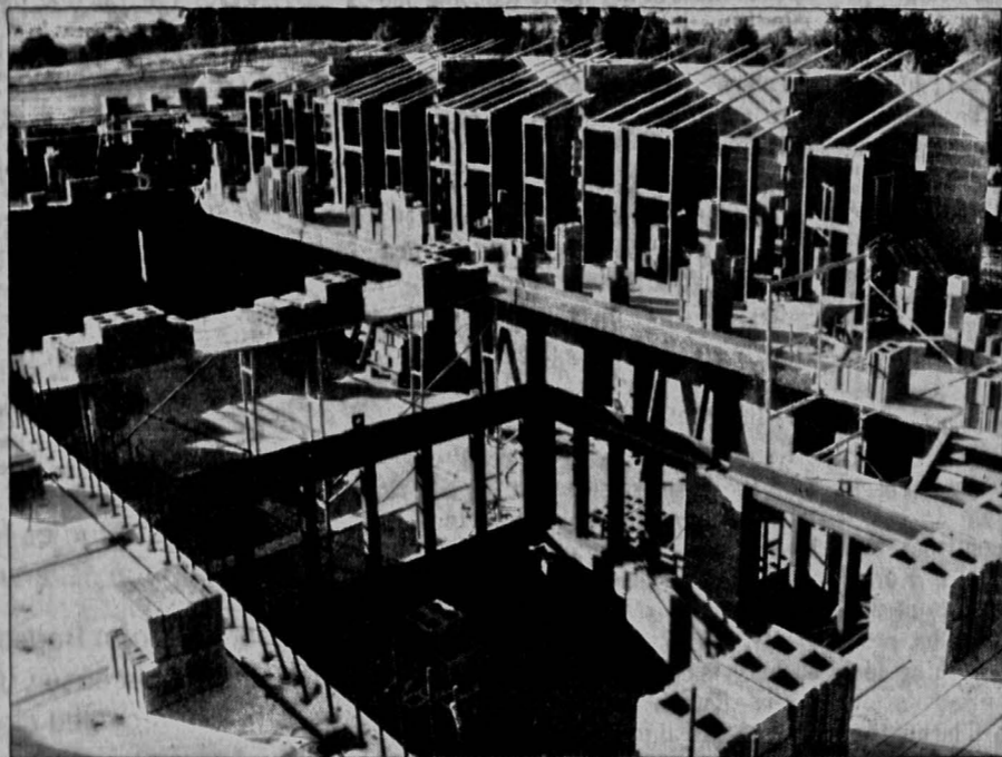
An unfinished cell block in the Iowa Security Medical Facility.
