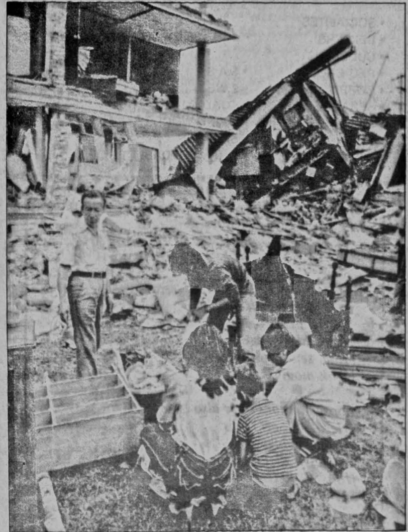
Members of a family in Popayan, Colombia collect their possessions Sunday after their home was destroyed by an earthquake. The quake hit the city Thursday and left at least 250 people dead, 1,500 injured and 100,000 left homeless.
