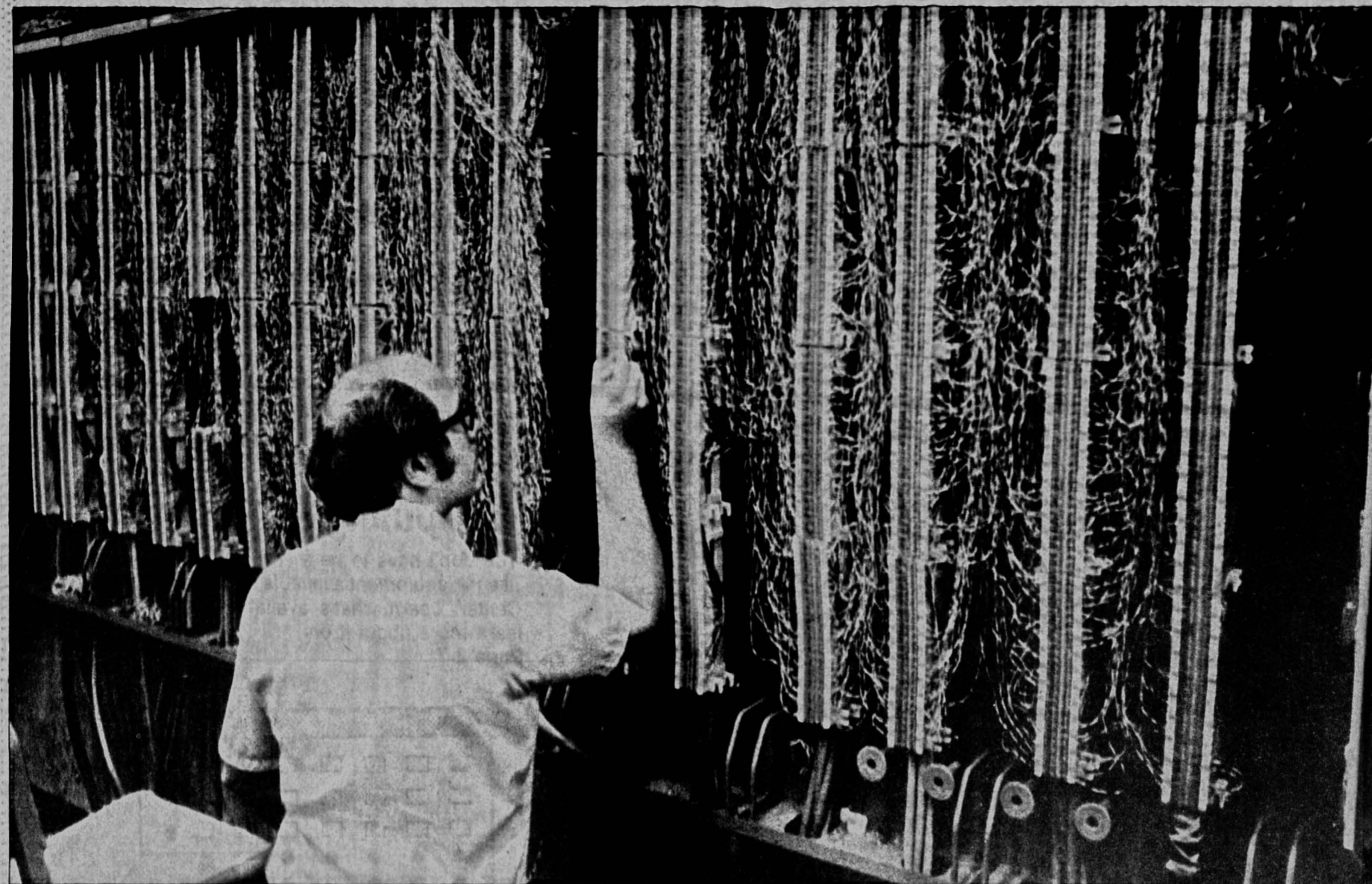
Electronic technician Jim Spahn connects some computer terminal circuits to telephone transmission wires in the Weeg Computing Center, in the basement of the Lindquist Center.
