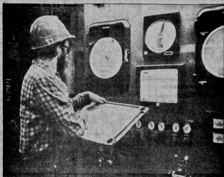
Taking steam gauge readings at the UI power plant.
