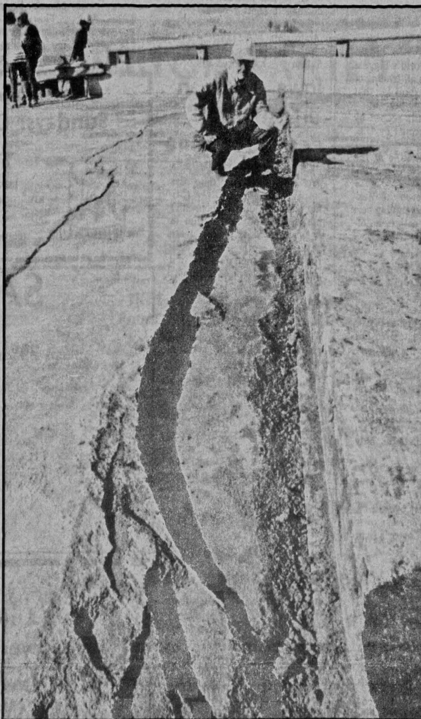
Left: Ervin Smitten, a California highway superintendent, inspects the dropped roadbed along Interstate 580.
