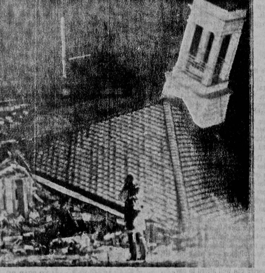
Police Station Wreckage The roof of the two-story Shaker Heights division police station in Cleveland ruts on the ground after an explosion early Monday but demolished the building. At least 15 persons were reported injured. The cause of the blast was not determined, but an official of the East Ohio Gas Co., of Cleveland, said it did not seem to be a gas explosion. — AP Wirephoto
