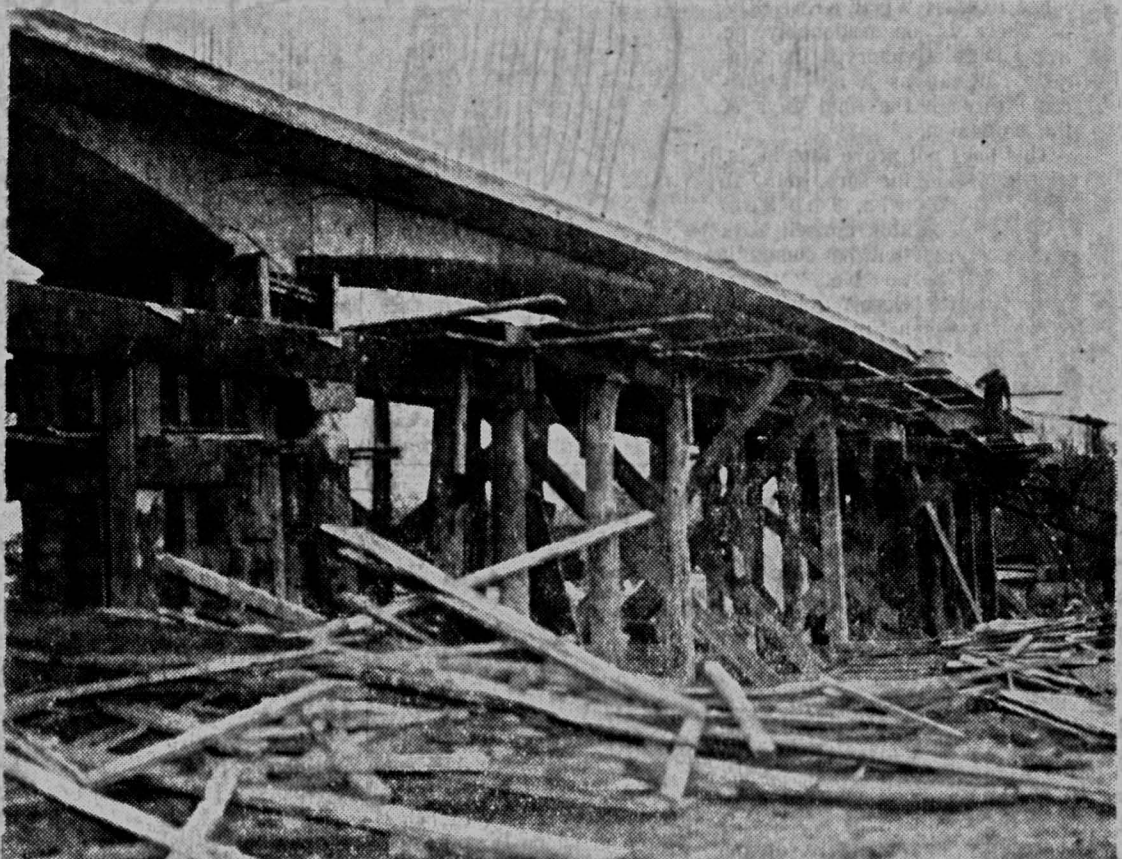
Overpass Nears Completion: Cement forms began to disappear on the new pedestrian bridge at the west end of the Iowa Avenue bridge Wednesday...
