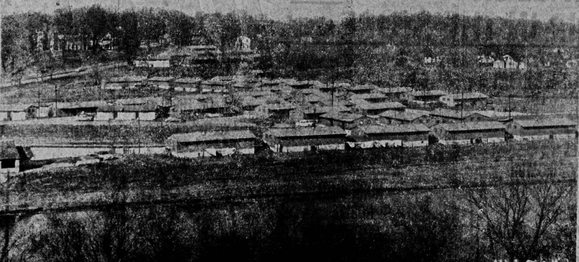
FROM THE EAST SIDE of the river the camera looks down on Riverside Park which houses 102 State University of Iowa married students and their families. One of nine housing developments which provide homes for 698 families, this unit was built in 1947 as a temporary measure. Riverside Park derives its name from its location on the Iowa River. (Photos by Art L. Davis.)
