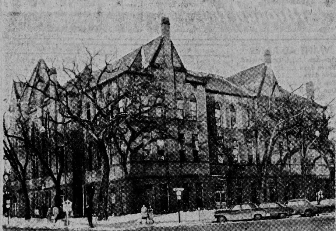
WHAT MANY STUDENTS BELIEVE to be the front of the 64-year-old Electrical Engineering building is actually the back. Through some confusion on the part of the builders, it was built facing north instead of south.
