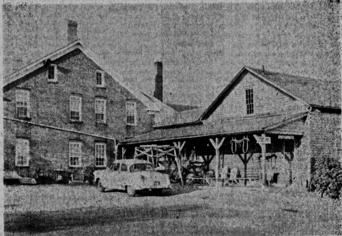
Back View & Parking Area
