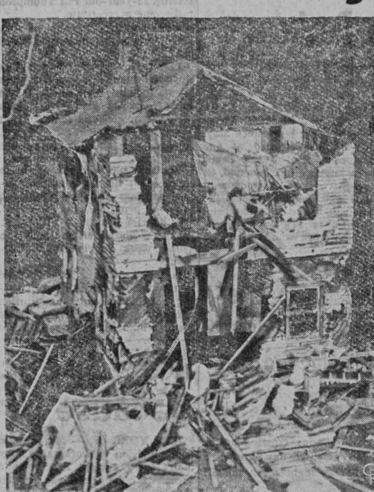
NEW WAY TO BUILD HOUSES! This is a scale model of the two-story wood-frame house built by civil defense for training courses.
