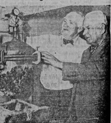
LATEST INVENTION of Dr. Lee DeForest who invented the vacuum tube so vital to radio broadcasting, is a machine to turn heat directly into electricity. Here he shows it to Dr. Robert Millikin (right) of California Institute of Technology, in Los Angeles. The idea somewhat resembles the vacuum tube. Dr. DeForest, 79, pumps air out of the metal pot (left), then a five-inch disc is heated to incandescence to throw off electrons.
