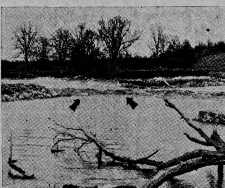
ARROWS POINT TO THE BREAK in the levee at the Iowa-Illinois Gas and Electric company dam in Coralville. Rising water and ice breached the levee shortly after midnight Friday. The levee was repaired with a rock and dirt fill last summer after being broken by the spring floods last year. Electric service was not impaired. (Daily Iowan Photo by Phyl White)
