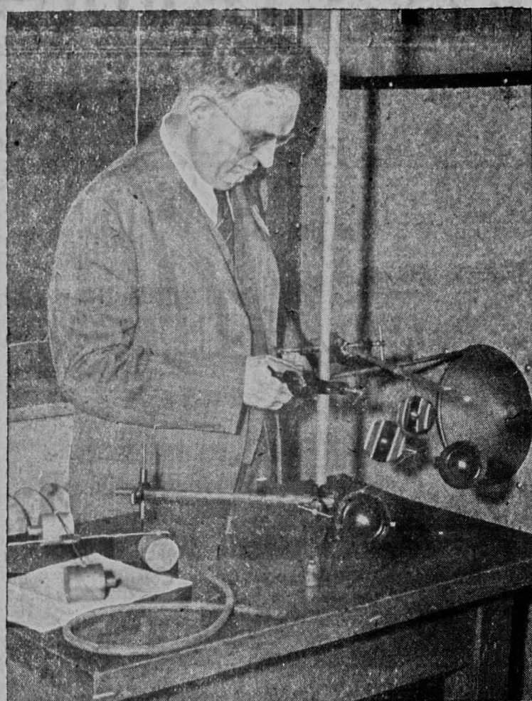
SOUND WAVES do the work in this acoustic reaction motor, one of 19 devices displayed by college physicists in an exhibit at the physics building last night. Constructed by two members of the Pennsylvania State college faculty, H.K. Schilling (above) and I. Rudnick, it demonstrates how mechanical energy can be obtained from sound waves. Waves from the speaker enter the spheres through the neck, and when air from the room meets the waves a resonance is set up. This blasts the air back through the neck and drives the sphere forward in a rocket-like manner.
