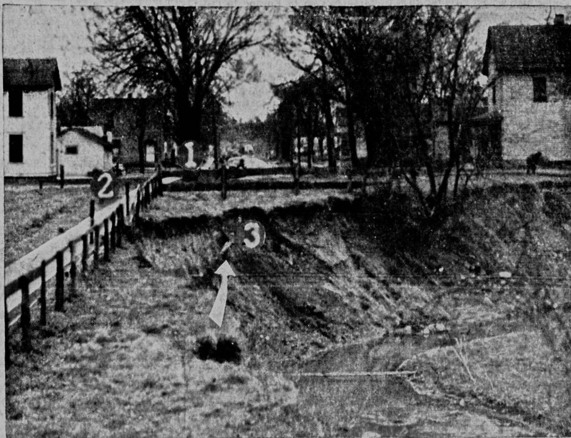
THERE USED TO BE A STREET where Ralston creek now rounds a bend across South Linn (1) near the Benton street bridge. But the street has gradually gone down the Iowa river via Ralston creek and erosion, and now a sidewalk bordering it (2) is also on the verge. Fence posts already have been undermined, menacing a railing along the embankment. Also exposed by erosion is an old gas main (3), long out of use. Acting upon city council direction, City Engineer Fred Gartzke last night submitted recommendations on how these and other defects can be remedied. A retaining wall would line the creek bed for 230 feet and permit restoration of Linn street. Investigating the problem is a special council committee composed of Alderman W.H. Grandrath (chairman), Clark F. Mighell and Max S. Hawkins.
