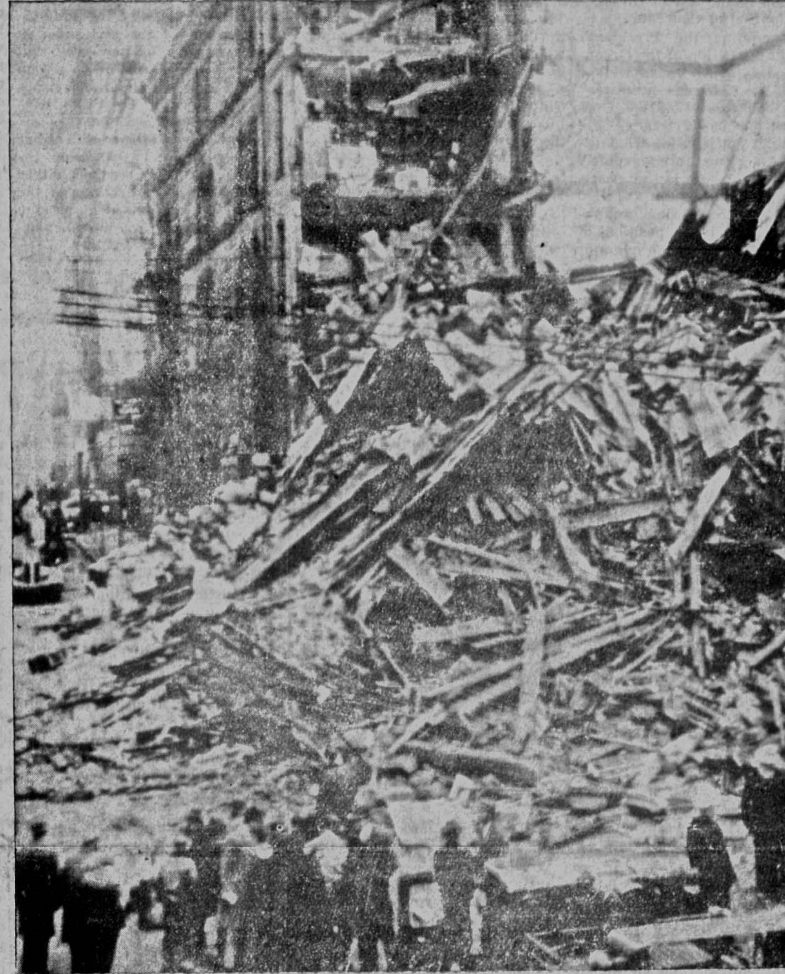
FOUR WORKMEN WERE TRAPPED when this five-story building collapsed in downtown Cincinnati yesterday. Hopes brightened late last night that three of the men would be crawled alive as firemen stepped up efforts to clear away the huge pile of rubble. A fireman said he had crawled into a "tunnel" in the wreckage and talked to one of the men. This man said he could hear two other men groaning. The whereabouts of the fourth man was unknown. (AP WIREPHOTO)
