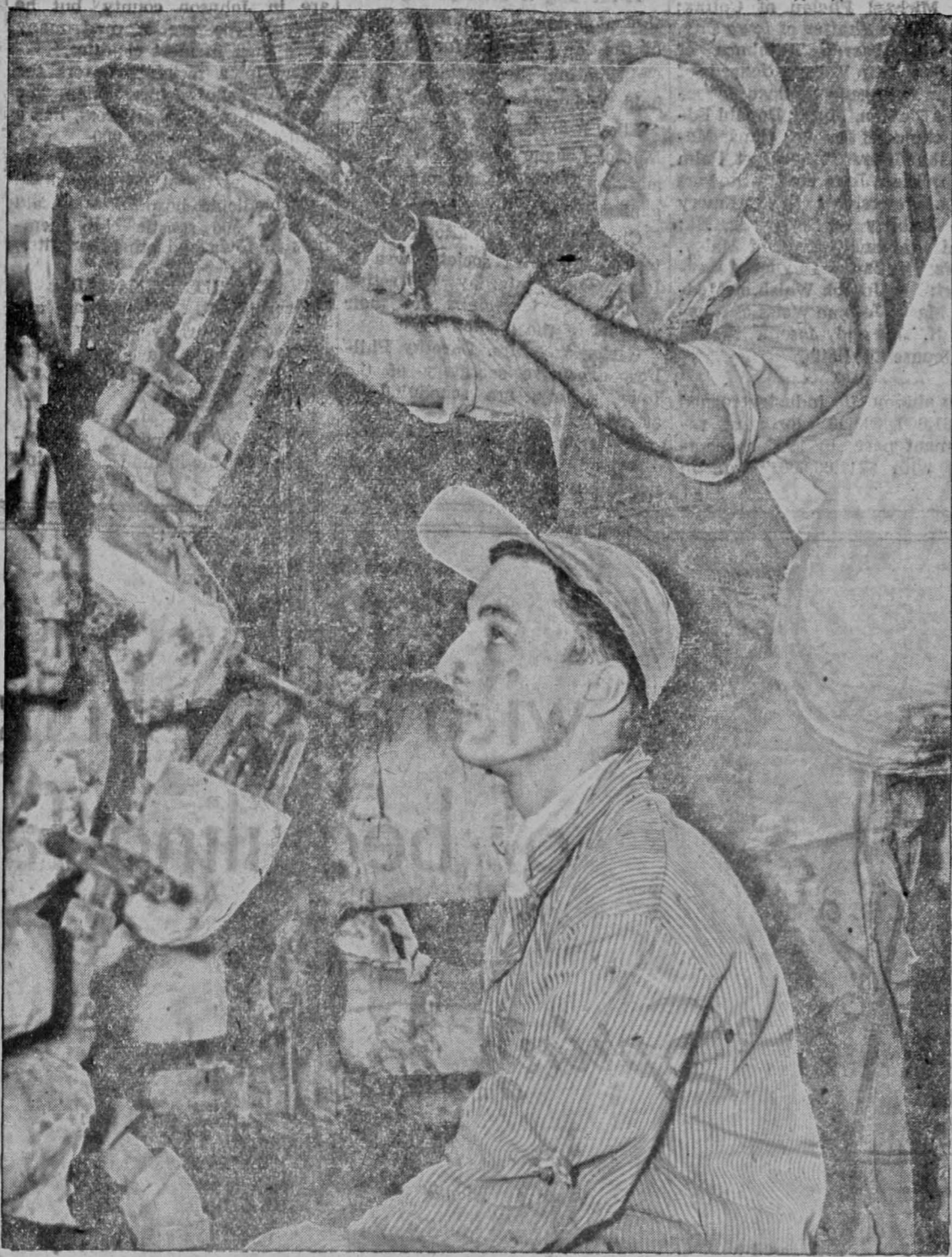
KEEPING A WATCHFUL EYE on a steam gauge, Cleo Stribley, 16 W. College street, kneeling, helps T. J. Parker, 1829 F street, steam fitter at the physical plant, regulate the flow of steam through the underground pipes of the university heating system. (Daily Iowan Photo by Dick Davis.)
