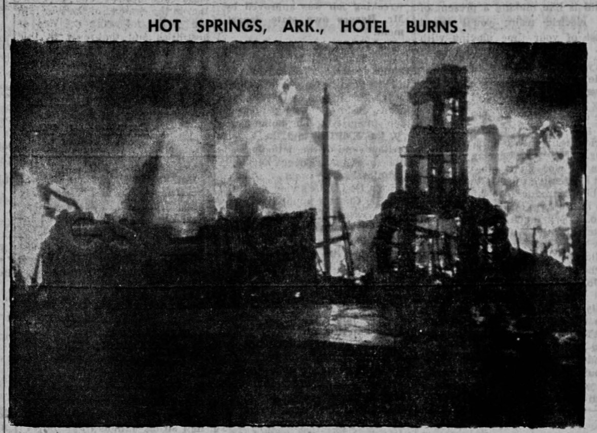
FLAMES ARE SHOWN sweeping the Great Northern Hotel in Hot Springs, Ark., early yesterday. The fire, discovered by a hotel porter about 1:10 a. m., leveled the 50-year-old, 75 room landmark. Although smoldering ruins delayed firemen searching for victims, it is known that at least one died and 10 were seriously injured. (AP Wirephoto)
