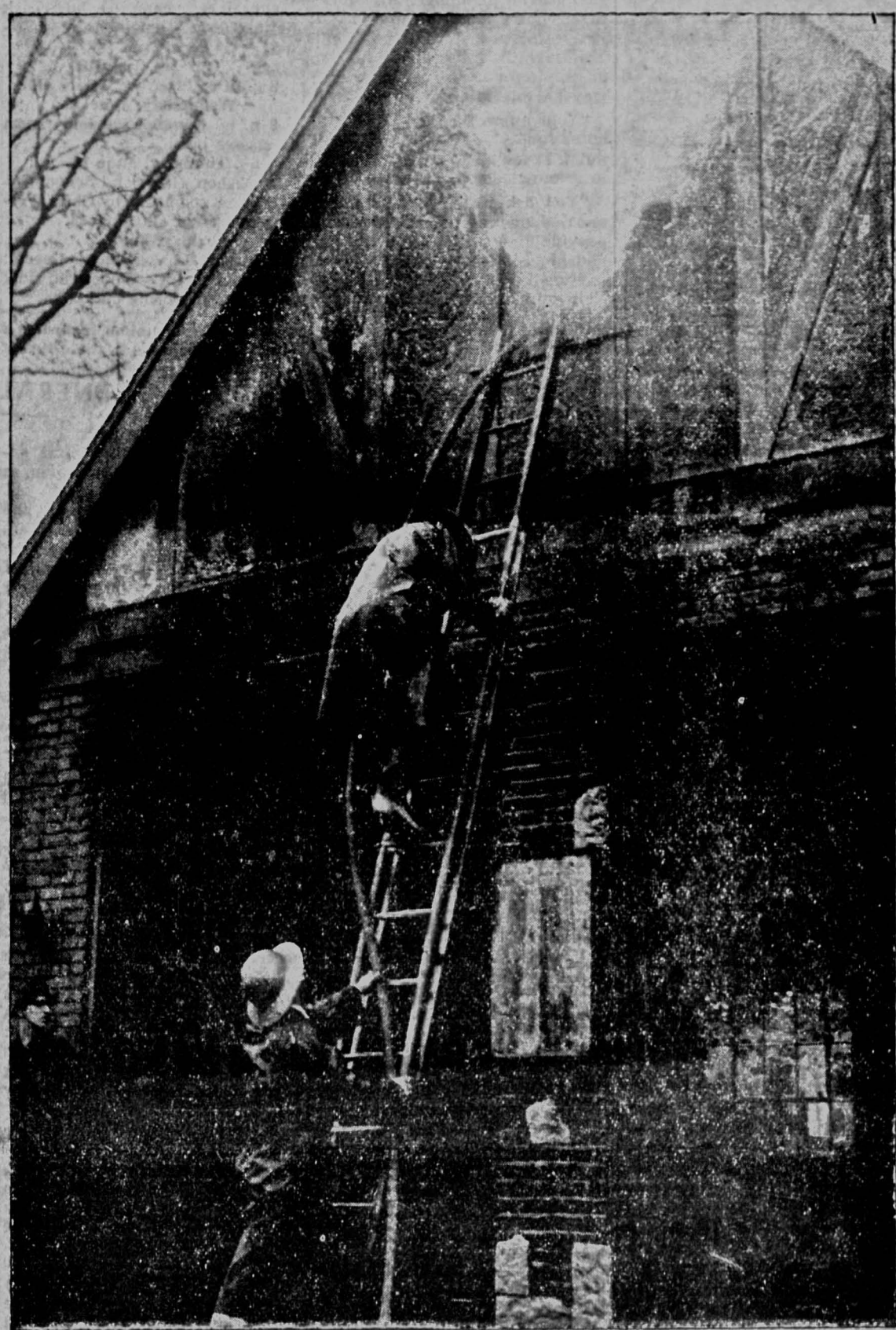
FIREMEN ARE shown climbing into the upper part of Bob and Henry's garage, 323 E. Burlington streets, to fight the fire that gutted the building yesterday afternoon. Resulting damage was estimated at $15,000 and Louis Goodwin, a Negro employee, was severely burned when his clothing caught fire. A gasoline tank on a truck and several barrels of anti-freeze exploded during the fire, making it extremely hazardous for firemen fighting the blaze. Fire Chief J. J. Clark said the fire was well started when firemen arrived but they quickly brought it under control. This same garage was damaged by a fire Jan. 14 when gasoline being used to clean the floor ignited. Story and picture on Page 6.
