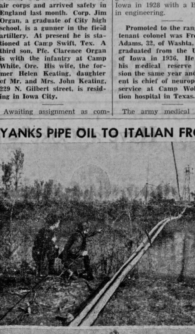
OIL PIPELINE constructed and put into operation in just one week insures a constant flow of precious oil to Allied forces on the Italian front. From its beginning at an Italian port the pipeline crosses a river, top photo, and finally terminates at a point near the front, bottom photo, where cans are being filled prior to distribution to various mobile outfits. (International)
