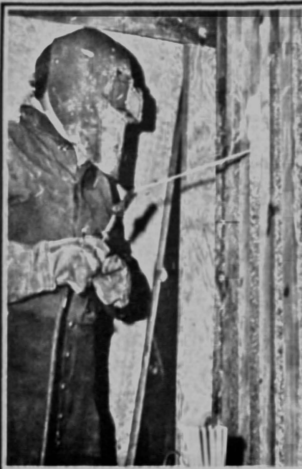
Welding plates for the tower.
