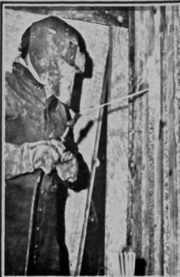
Welding plates for the tower.
