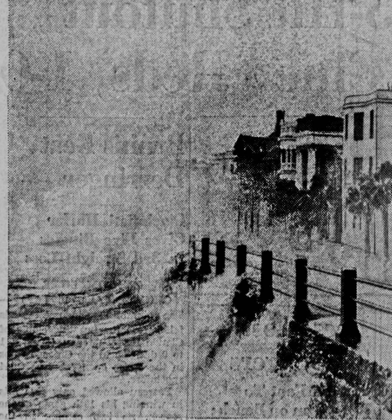
The fury of the tropical hurricane that ripped along the South Carolina coastline is seen in this photo of a seawall at Charleston being battered by tremendous waves that accompanied the 100-mile per hour winds. Many coastal areas were flooded by accompanying high tides. Property damages were heavy but few lives were lost, according to early reports.
