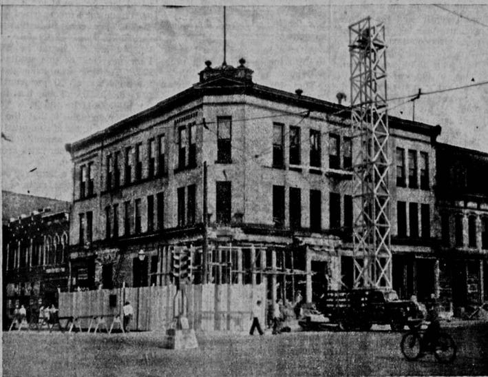
A hoisting tower has been erected beside the old Iowa City Savings bank building, above, as work progresses in demolishing the structure to replace it with a \$100,000, three-story structure housing 30 offices and other concerns. Only a shell now remains of the building, most of the in-
