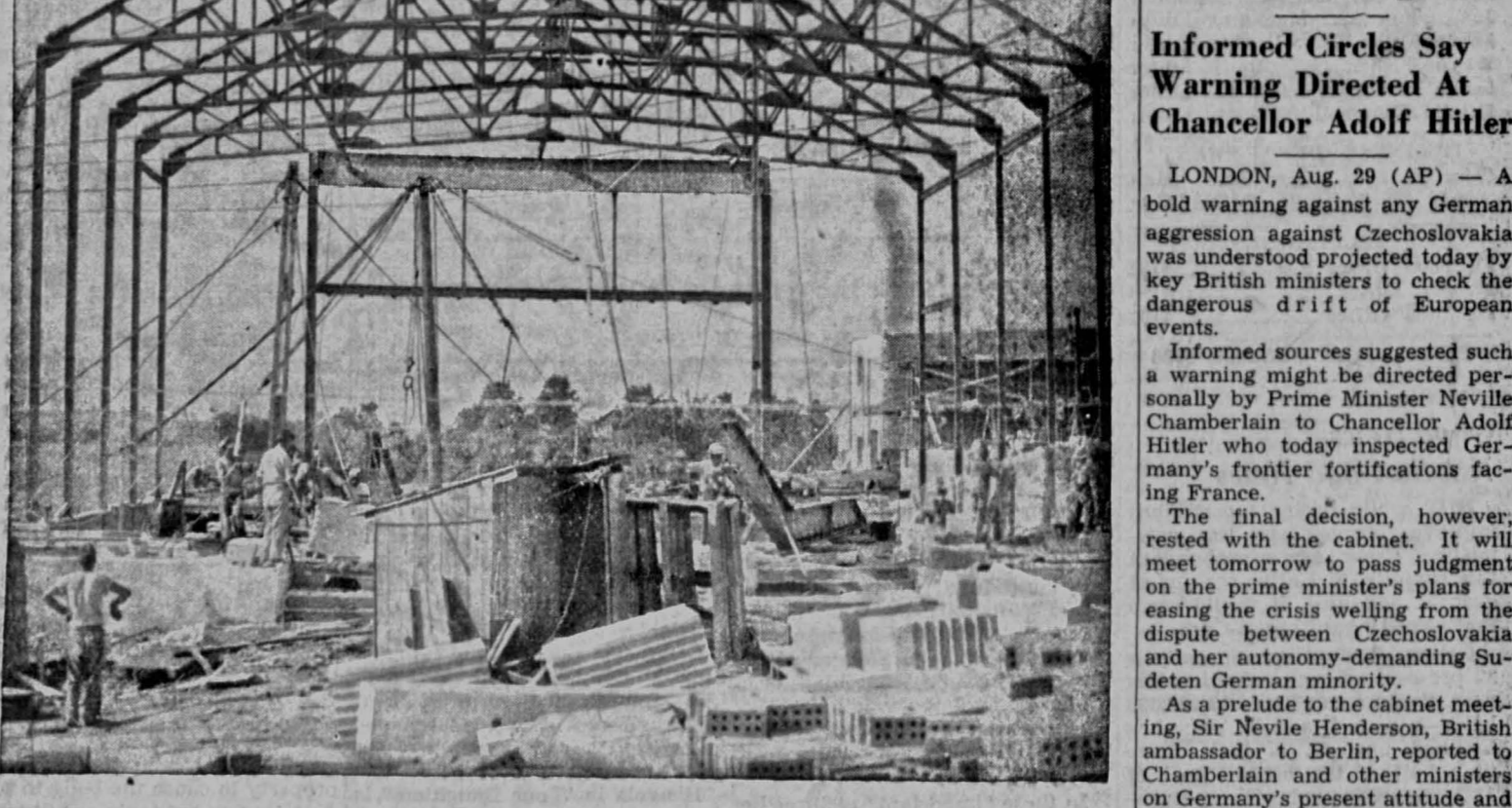
Shakespeare may have exaggerated, but this is a stage—or will be. It's the auditorium of the new Iowa City high school building, costing $725,000 and rapidly taking shape in Morningside addition, east Iowa City. The walls of the building are now being built, and part of the roof will be on by the time snow flies.
