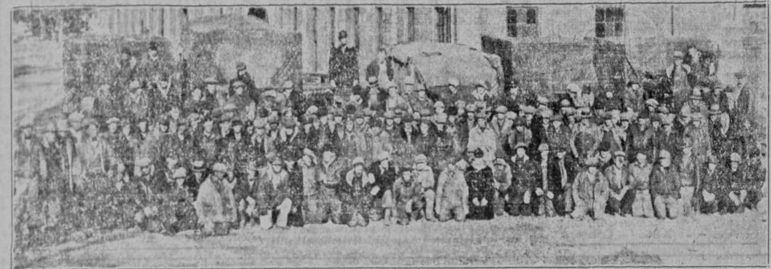
These men constitute one of the two shifts of 100 men each who are employed in constructing a natural gas pipe line from Ainsworth to Cedar Rapids. With the exception of foreman and engineers, all the men are residents of Iowa City, formerly unemployed. The acquired their jobs through the influence of the Iowa City Light and Power company, whose parent organization, the United Light company, is building the line.
