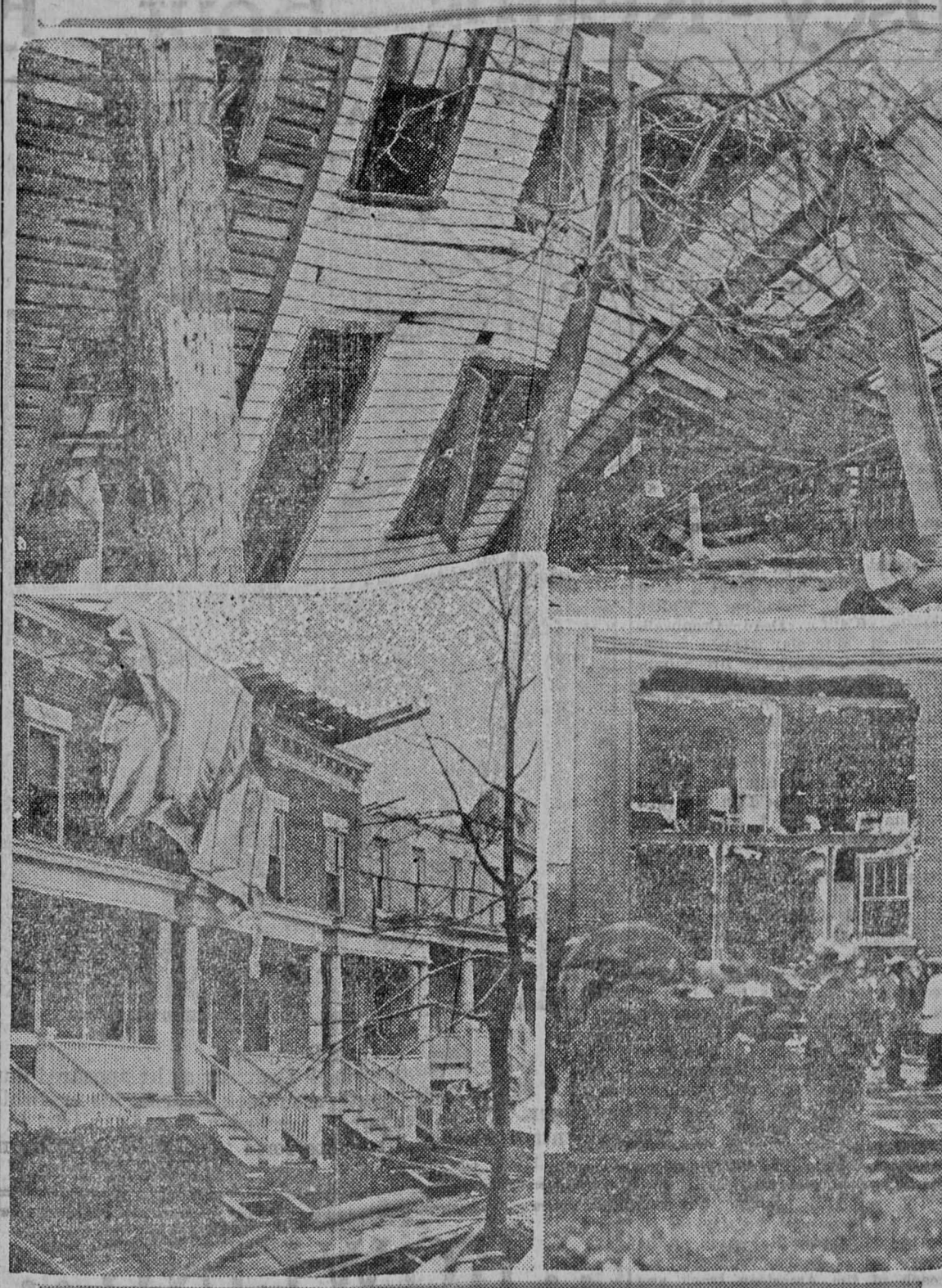
Upper photo shows how twister ripped several homes in Washington. Lower left: View of 14th street, showing destruction in path of storm. Lower right: The Noel School after being struck by terrific gale.
