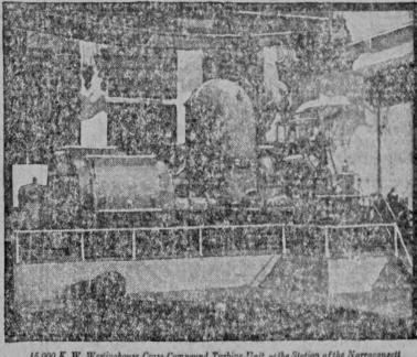
Equally impressive, oil was pumped through the self-contained lubricating system to the bearings at the rate of 600 gallons a minute. Had the oiling system failed for only 30 seconds, the bearings would have been wrecked, and other parts of the unit harmed!
