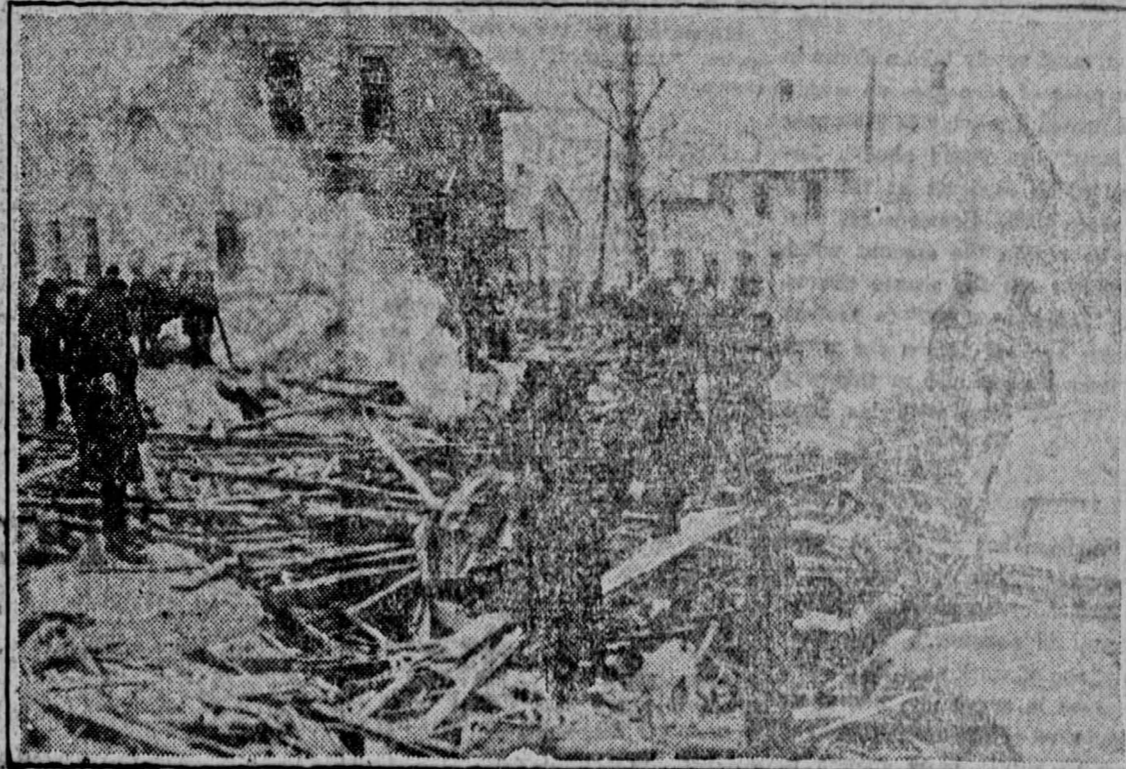
Ruins of the house at Manville, R. I., in which 15 were killed by a gas explosion
