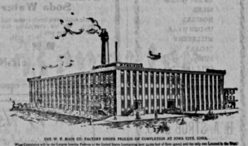
THE W. F. MAIN CO. FACTORY UNDER PROCESS OF COMPLETION AT IOWA CITY, IOWA. Plans Containments will be the Largest Jewelry Factory in the United States (containing over 1,000,000 sq. ft. of floor space) and the only one located in the West!
