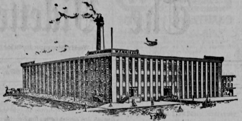
THE W. F. MAIN CO. FACTORY UNDER PROCESS OF COMPLETION AT IOWA CITY, IOWA. When Completed will be the Largest Jewelry Factory in the United States (containing over 55,000 feet of floor space) and the only one Located in the West.
