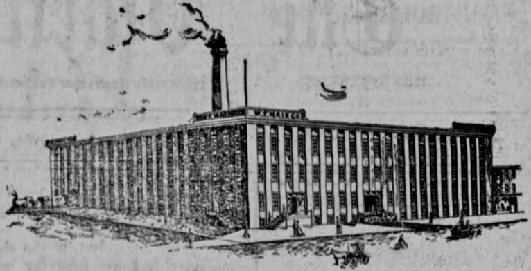
THE W. F. MAIN CO. FACTORY UNDER PROCESS OF COMPLETION AT IOWA CITY, IOWA. This considered will be the largest jewelry factory in the United States (containing over 55,000 feet of floor space) and the only one located in the West.
